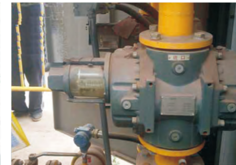
Gas roots flowmeter in gas mixture field
